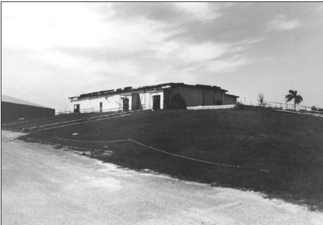
**Plate 115. SAC alert. Oblique view of berming for the molehole at the former Homestead Air Force Base, 1995. Courtesy of Mariah Associates, Inc.**
