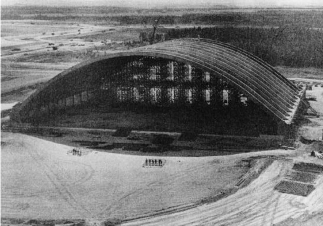
**Plate 10.** Anton Tedesko, Roberts & Schaefer. Construction, B-36 hangar at Loring Air Force Base, September 1948. Reproduced from *Army Engineers in New England* (1978).
