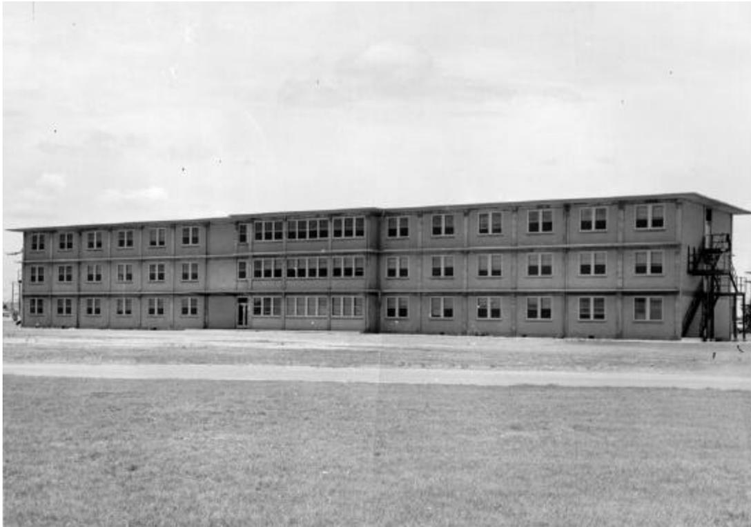
**Plate 78. Concrete-block airmen dormitory, with three-man rooms. Bergstrom Air Force Base. 1952-1953. Courtesy of the Air Force Historical Research Agency.**
