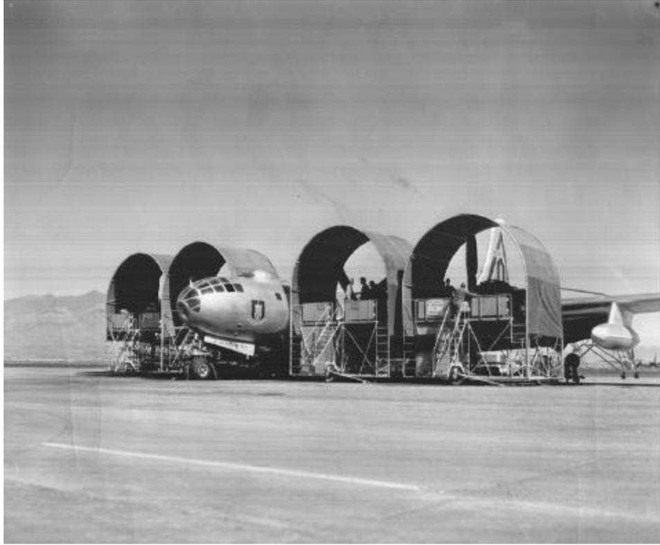
**Plate 55. Moveable repair docks for the engines of the B-50. Biggs Air Force Base. 14 September 1951. Courtesy of the Air Force Historical Research Agency.**
