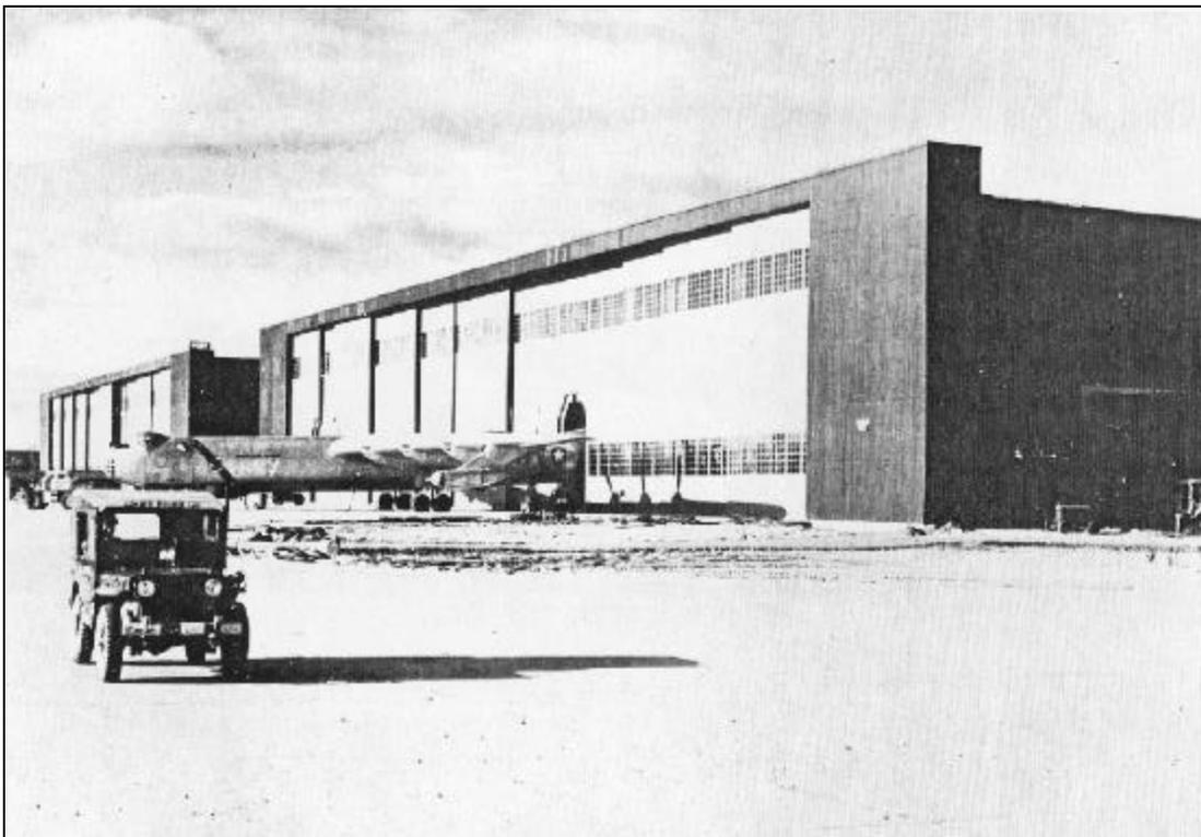
**Plate 31. Kuljian Corporation. Paired, medium bomber (two-bay) double-cantilever hangars at Goose Bay Air Base. View of the middle 1950s. Courtesy of the Kuljian Corporation.**
