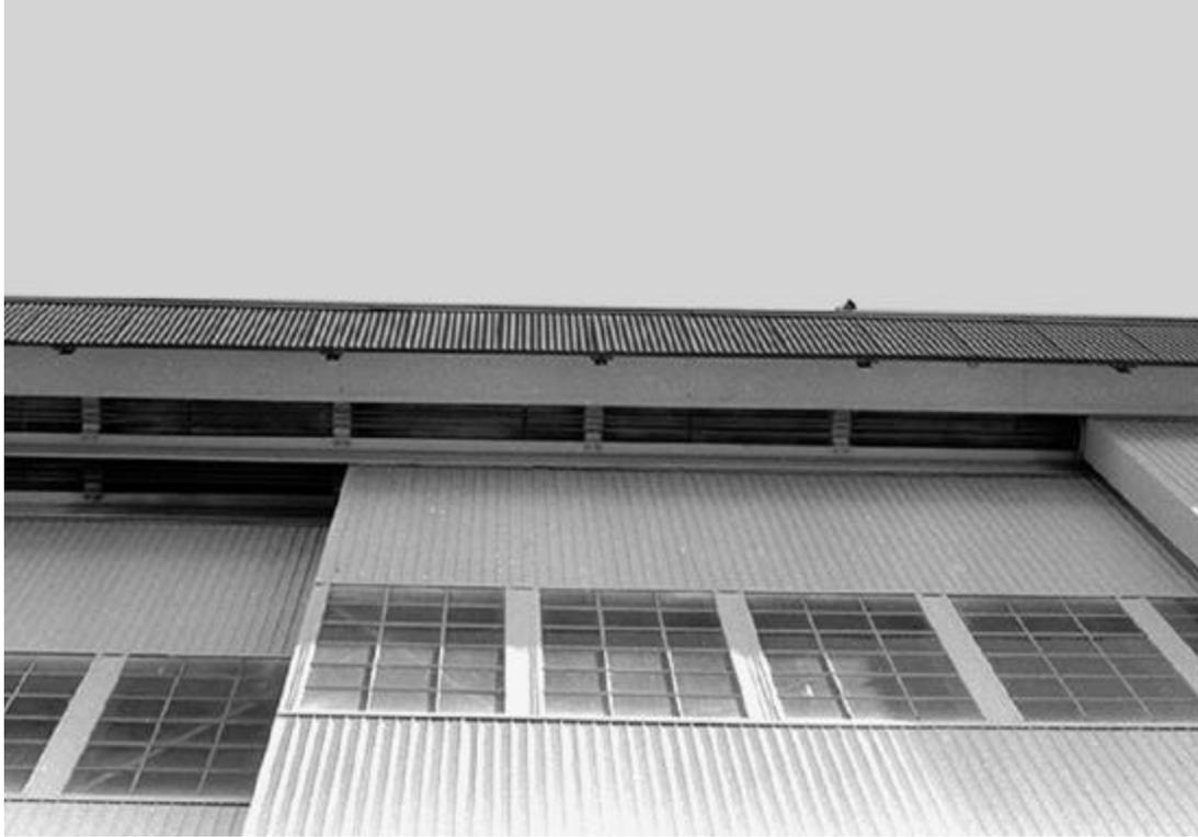
**Plate 41. Upper tracks for recessing doors. Double-cantilever hangar at the former Mather Air Force Base. View of 1998. Photograph, K.J. Weitze.**
