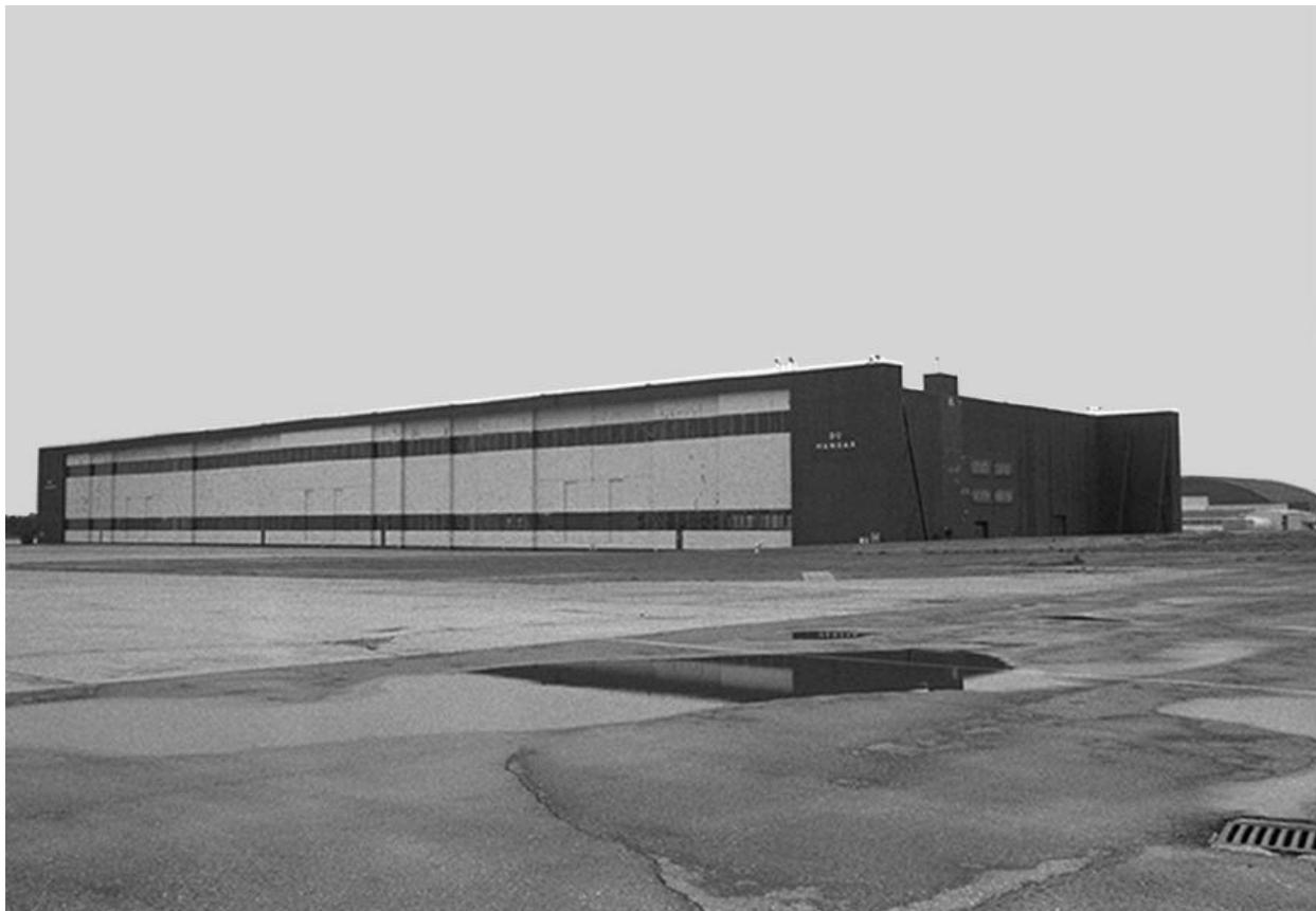
**Plate 29. Kuljian Corporation. Heavy bomber (three-bay) double-cantilever hangar at the former Loring Air Force Base. View of 1995. Courtesy of Mariah Associates, Inc.**
