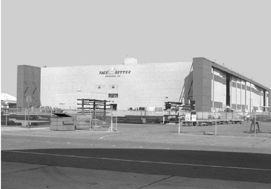
**Plate 32. Kuljian Corporation. Heavy bomber (three-bay) double-cantilever hangar at the former Castle Air Force Base. View of 1998. Photograph, K.J. Weitze.**
