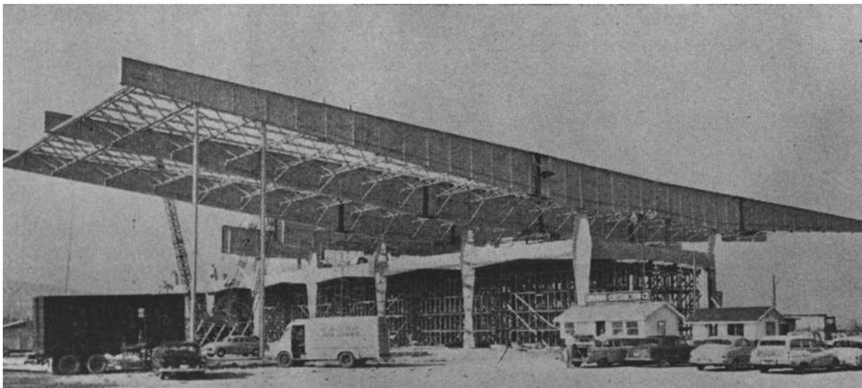
**Plate 45.** Skidmore, Owings & Merrill. Cantilever construction for United Airlines hangar, San Francisco International Airport. *Engineering News-Record*. 30 January 1958.
