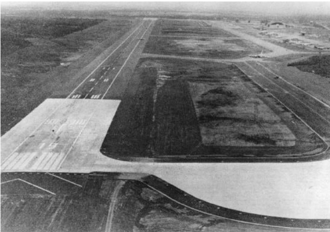
**Plate 86. Reinforced concrete overruns (1000 feet) and warm-up pads, 21 inches thick. Added, Loring Air Force Base, 1956. *Engineering News-Record*. 28 February 1957.**
