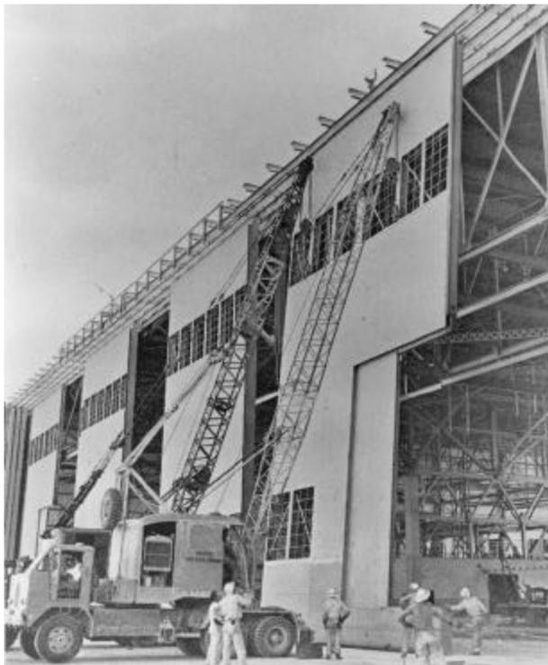
**Plate 40. Construction for recessing doors. Double-cantilever hangar program. Courtesy of Kuljian Corporation.**
