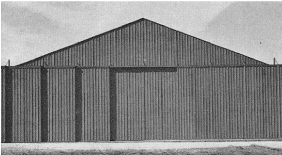
**Plate 54.** Butler Manufacturing. Prefabricated hangar for the Army Air Forces, with steel doors and roof. 1945. *The Military Engineer*. May 1945.
