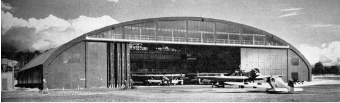
**Plate 5. Dyckerhoff & Widmann. Thin-shell concrete hangar completed outside the U.S.
