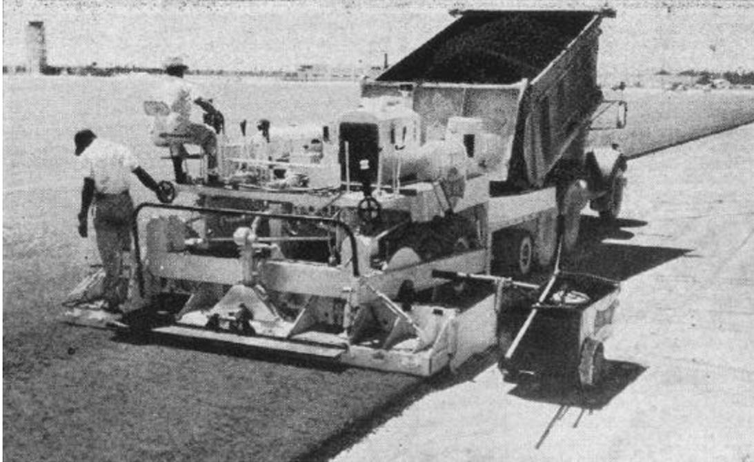
Plate 87. Paver laying tar-rubber surface resistant to jet fuel and blast damage. Homestead Air Force Base. *Engineering News-Record*. 16 June 1955.
