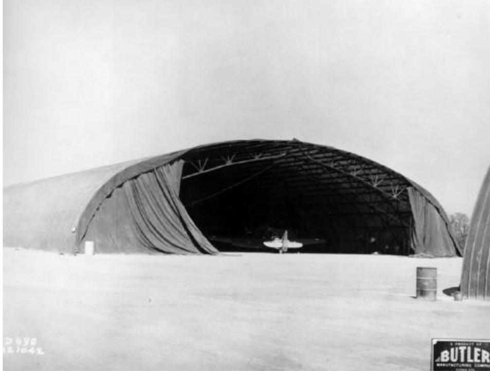
**Plate 49. Butler Manufacturing. Canvas-covered hangar for the Army Air Forces. 1942. Courtesy of the Butler Manufacturing Company.**
