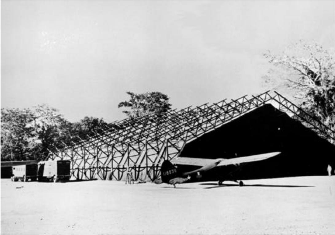
**Plate 51. Butler Manufacturing. Combat hangar, type CH, erected at Espiritu Santo, New Hebrides, Army Air Forces. 1942. Courtesy of the Butler Manufacturing Company.**
