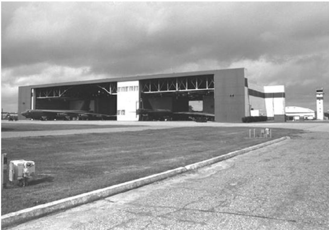
**Plate 42. Kuljian Corporation. Basic double-cantilever hangar at Barksdale Air Force Base. View of 1995. Courtesy of Mariah Associates, Inc.**
