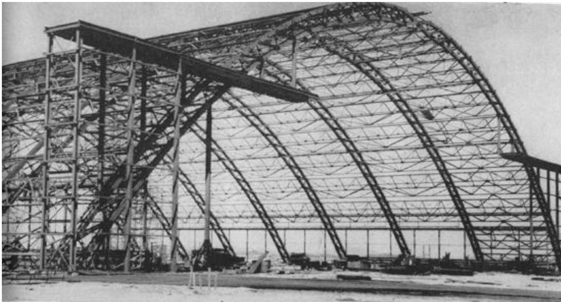
**Plate 43. Construction for test hangar at Edwards Air Force Base. *Engineering News-Record*. 9 August 1956.**
