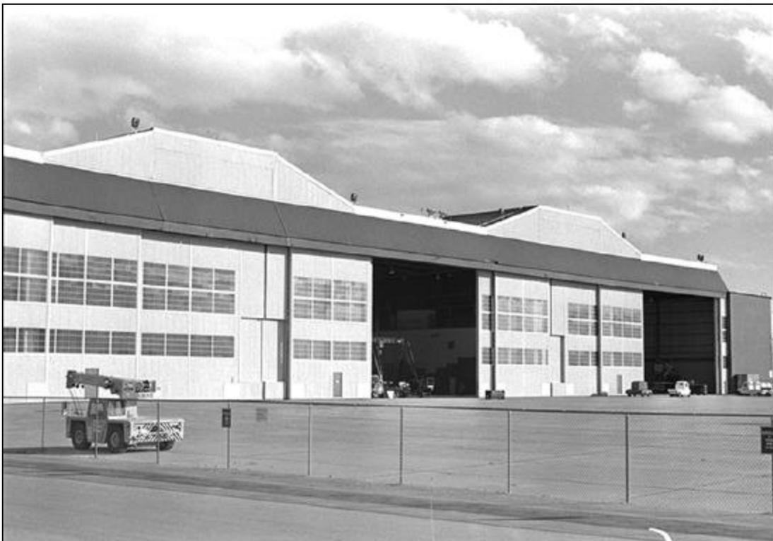
**Plate 24. Mills & Peticord. Double-cantilever hangar at Kirtland Air Force Base. View of 1998. Photograph, K.J. Weitze.**
