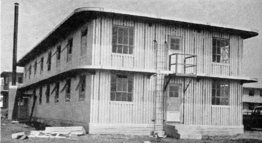
**Plate 76.** Holabird & Root. Experimental steel dormitory (two of this design built). Camp Grant, Illinois. *Engineering News-Record*. 22 May 1941.
