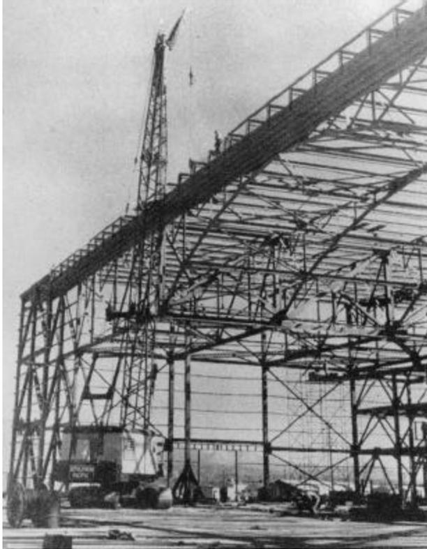
**Plate 39. Double-cantilever hangar under construction at March Air Force Base. *Engineering News-Record*. 12 May 1955.**
