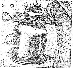
INSTALLATION OF DOME LIFTING HANDLE IN BESTHER HOLE
