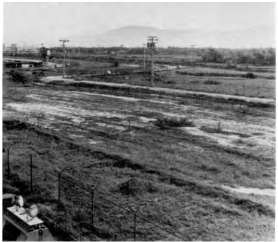
A portion of the double cyclone fence installed around the perimeter of Da Nang Air Base
