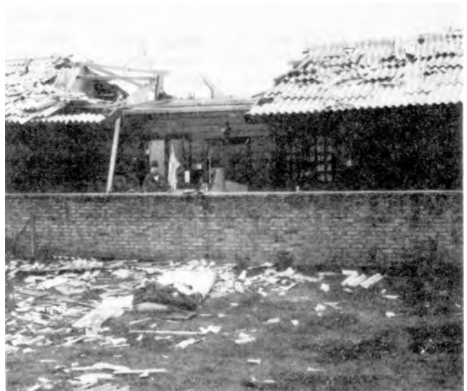
Brick revetments constructed about billets at Pleiku Air Base to protect against shell fragments. Such revetments were useless against direct hits
