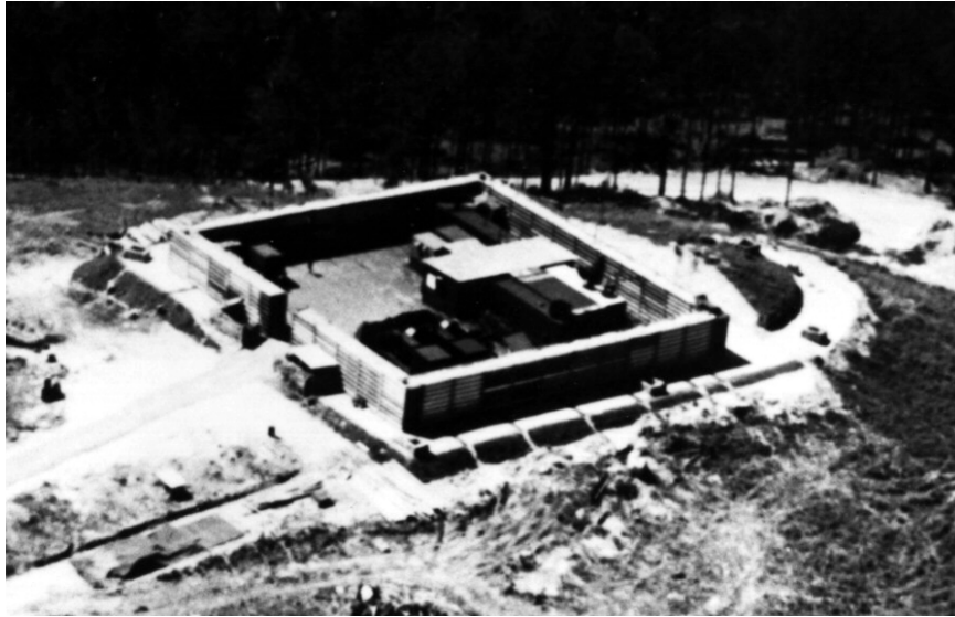
Combat Skyspot installation at Da Lat, South Vietnam.
