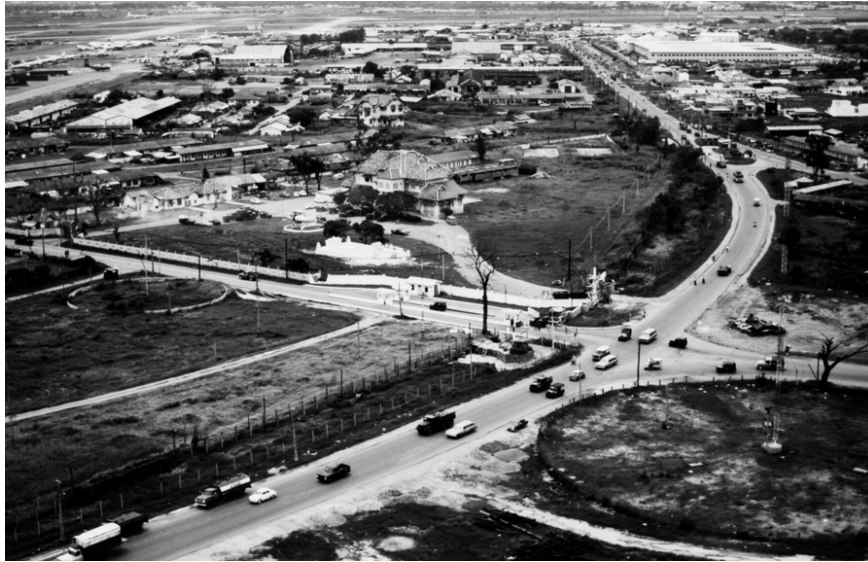
Gates to Tan Son Nhut, showing proximity of base to city.
