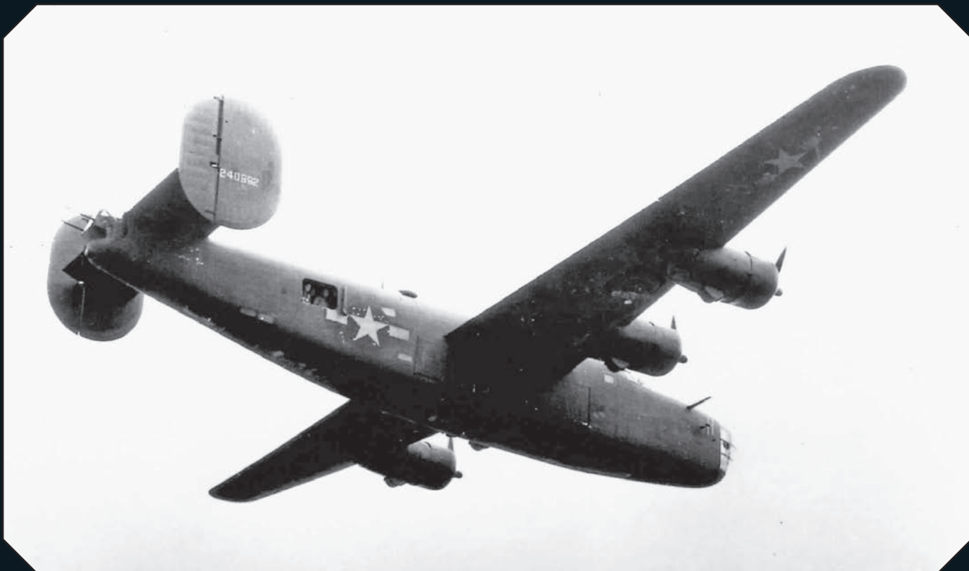
Bulges of flame-hiders cover engine exhausts on this black CARPETBAGGER B-24D. (Photo courtesy of the Moore Collection)
